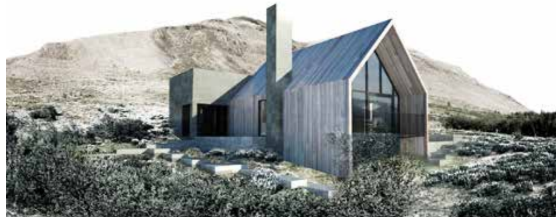
HELGI STEINAR HELGASON, ARCHITECT A single-family home for an elderly couple in the countryside of Kjós in South Iceland. The simple shape is inspired by the surrounding landscape: barren mountains and typical heather vegetation. The main building material is traditional Icelandic concrete, cast in situ and clad with local spruce panels. Construction is scheduled to be finished autumn 2015.
