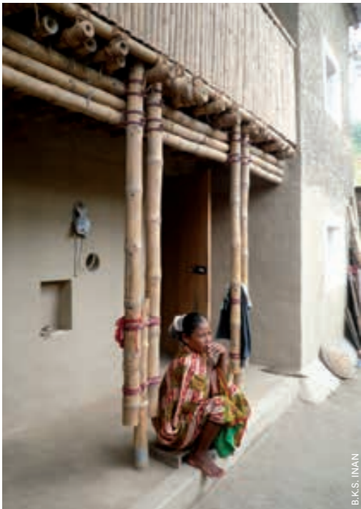
↑ HOMEmade in Rudrapur, Bangladesh, comprises three two-storey dwellings with living room, bedroom, storage space and veranda, built with clay and straw bricks (Studio BASEhabitat, Kunstuniversität Linz).
