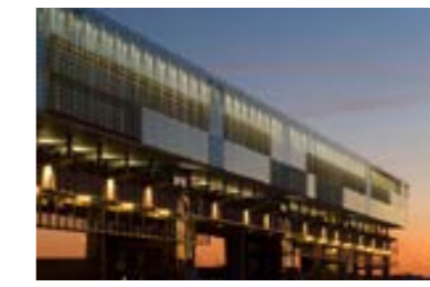
15 CRANE TRACK OFFICE BUILDING (1952, 2007) Architect: OTH architecten (Trude Hooikaas, Julian Wolse, Steven Reisinger, Gerald Lindner) Address: Kraanspoor 12-58 Info: www.oth.nl
