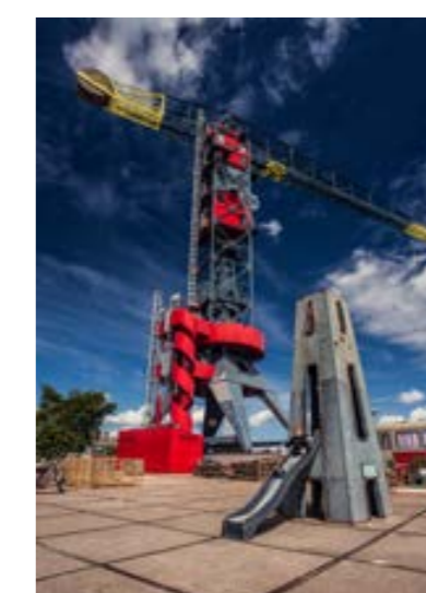
16 NDSM CRANE HOTEL (2014) Architect: IAA Architecten Address: NDSM-Plein 78 Info: www.iaa-architecten.nl
