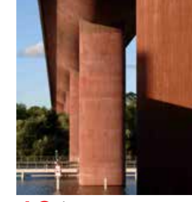
19 ÅRSTA BRIDGE (2005) Architect: Foster + Partners Address: Tantogatan 75
