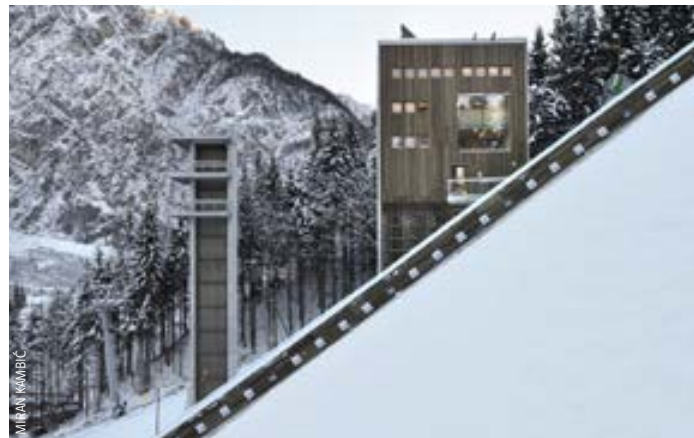
↑ The recently completed Nordic Ski Centre in Planica by A.biro symbolically represents making a leap in architecture, culture, sport and development.
