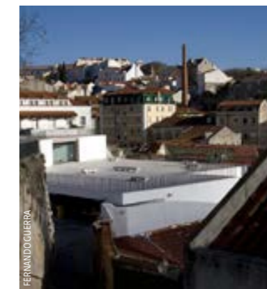
15 PORTAS DO SOL PARKING AND SQUARE (2006) Architect: Aires Mateus Address: Rua de São Tomé, Lisbon
